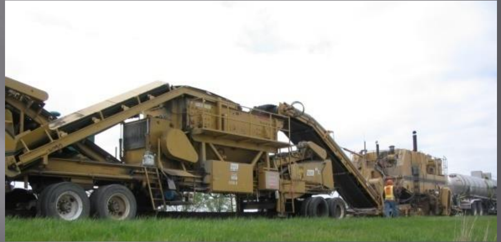
Cold In-Place Recycling
