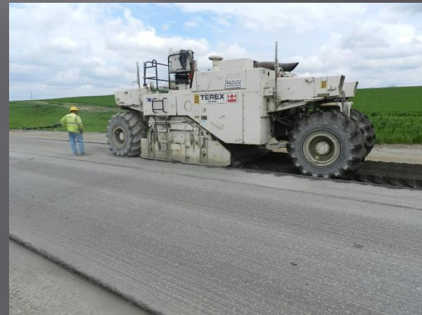
Full Depth Reclamation
